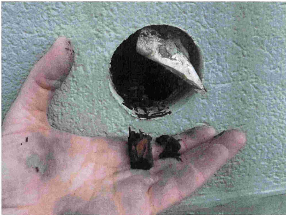
EXPLORAYORY OPENING #4 – SOUTH ELEVATION, PARAPET INTERFACE
