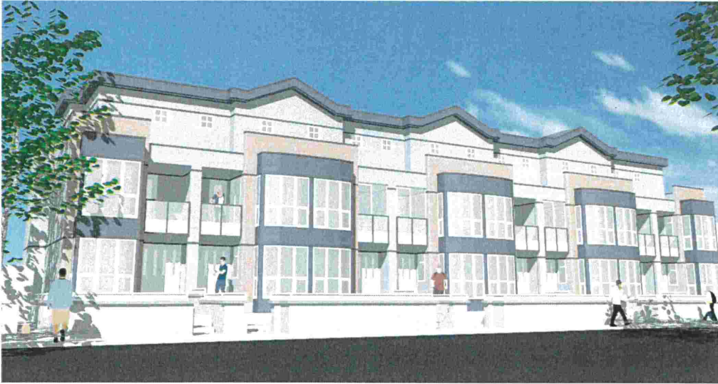
Figure 3.29 Existing colour scheme is renewed, new cross-cavity flashing and metal cap flashings are installed with a contrasting charcoal colour. Balcony guardrails match the colour of metal flashings and incorporate full height guardrails with privacy glass and clear glass panel guardrails.
