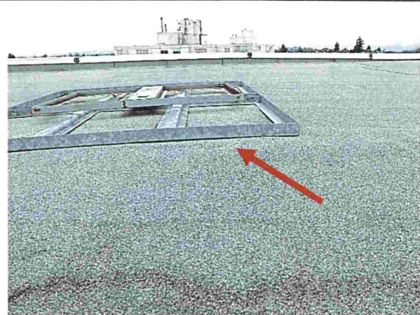
Photograph 45: Mechanical Penthouse The arrow points to metal debris on the rooftop.
