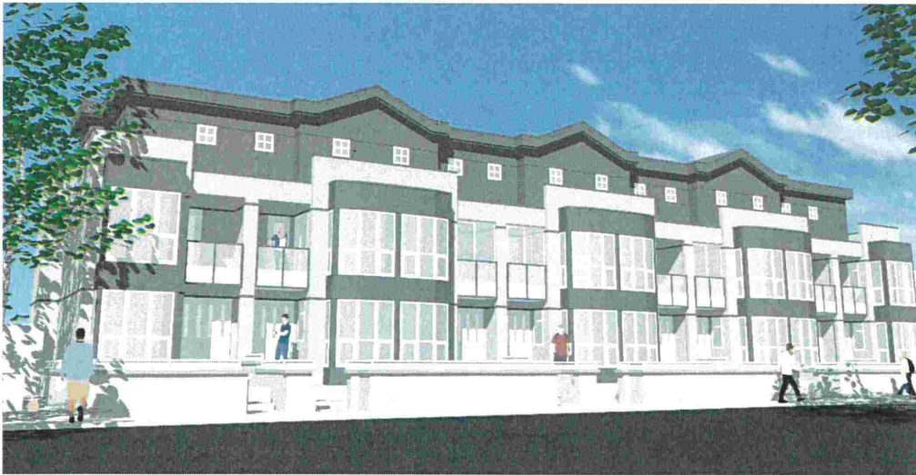
Figure 3.31 Pastel Green colour scheme with charcoal accents. New cross-cavity flashing and metal cap flashings are installed with a charcoal colour. Balcony guardrails match the colour of metal flashings and incorporate full height guardrails with privacy glass and clear glass panel guardrails.
