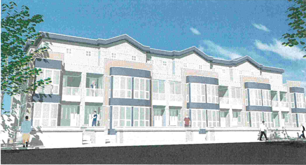
Figure 3.28 Existing colour scheme is renewed, new cross-cavity flashing and metal cap flashings match the colour of the existing metal flashings. Balconies incorporate full height guardrails with privacy glass and clear glass panel guardrails.
