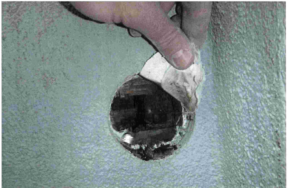
EXPLORAYORY OPENING #5 – SOUTH ELEVATION, DECK DIVIDER WALL
