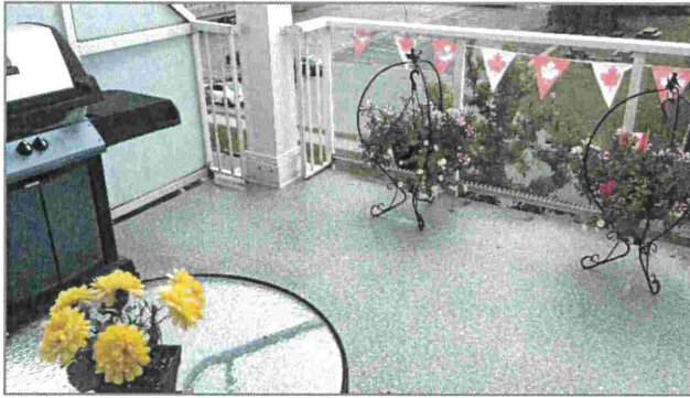
Figure 3.7 Example of a vinyl membrane on a wood substrate. Note: This photo is not from Joyce Place.
