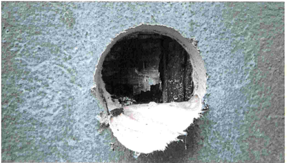
EXPLORAYORY OPENING #3 - EAST ELEVATION, WINDOW INTERFACE
