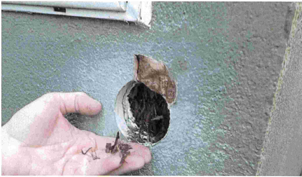
EXPLORAYORY OPENING #2 - EAST ELEVATION, WINDOW INTERFACE
