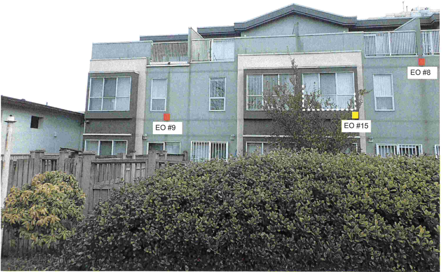
SOUTH ELEVATION, WEST END
