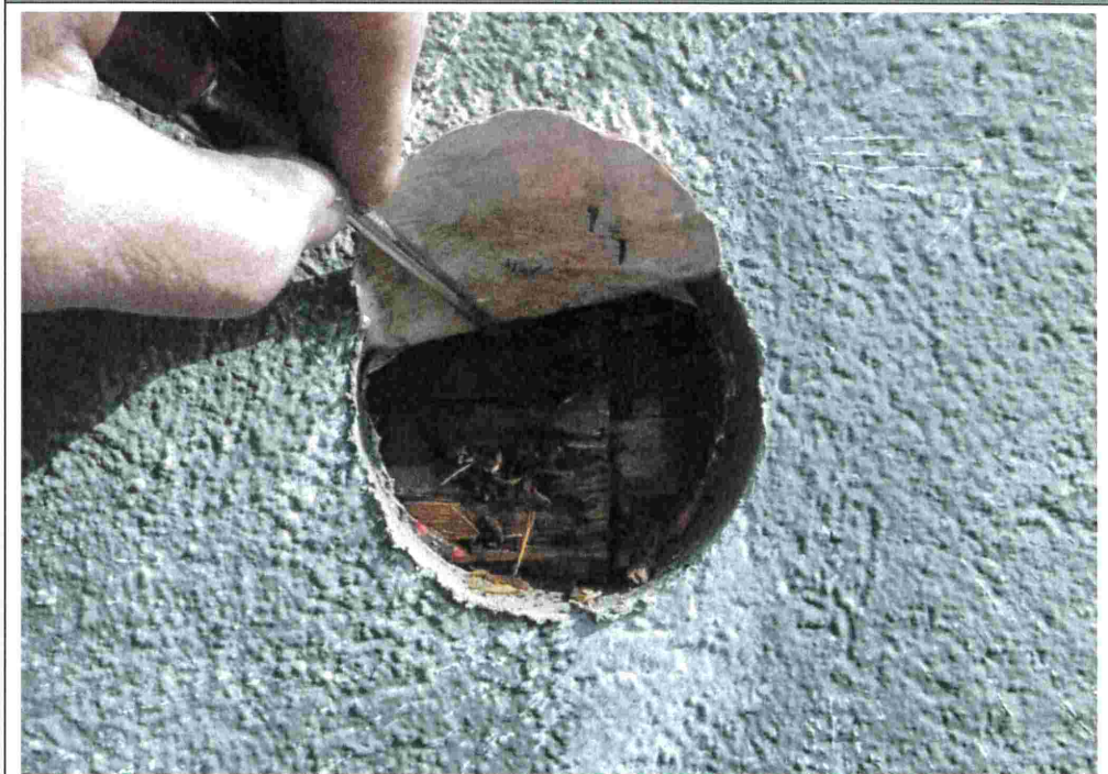
EXPLORAYORY OPENING #7 – SOUTH ELEVATION, WINDOW INTERFACE
