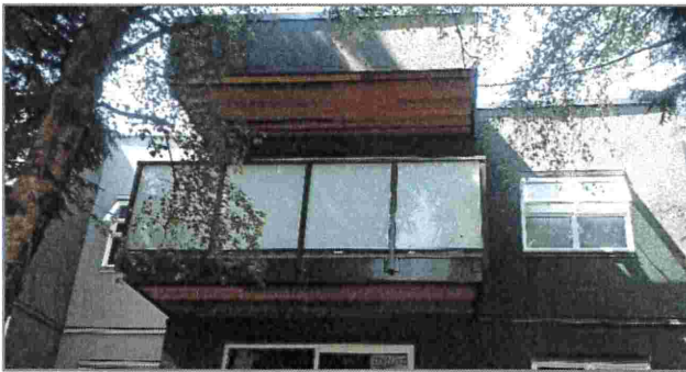
Figure 3.10 Aluminum-framed guardrail with opaque glass.
