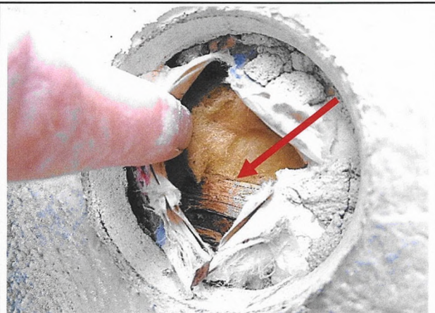
Photograph 53: Town Homes (#3376) EO made at the narrow wall facing South at floor level 2, below a horizontal joint. The arrow points to decayed plywood sheathing board.
