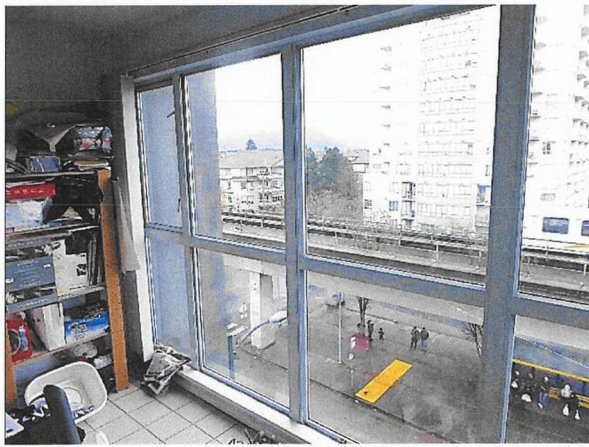
Photograph 9: Tower View of a typical "window wall" at an enclosed balcony (North elevation).
