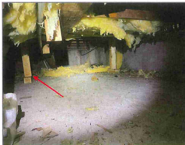
Figure 4 Unit 3376 - Crawl space. Out of plumb post not fully bearing on the supporting plate (red arrow).
