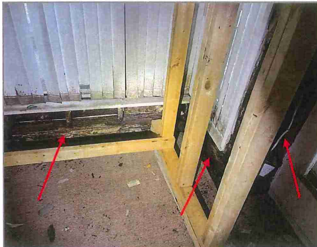
Figure 3 Unit 3376 - Deteriorated exterior wall - main floor
