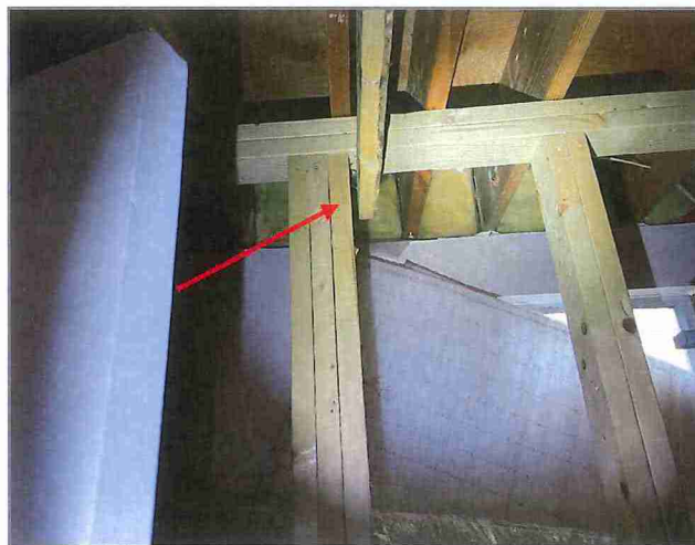
Figure 1 Unit 3362 – Main floor shoring The arrow indicates the location of a loose brace.
