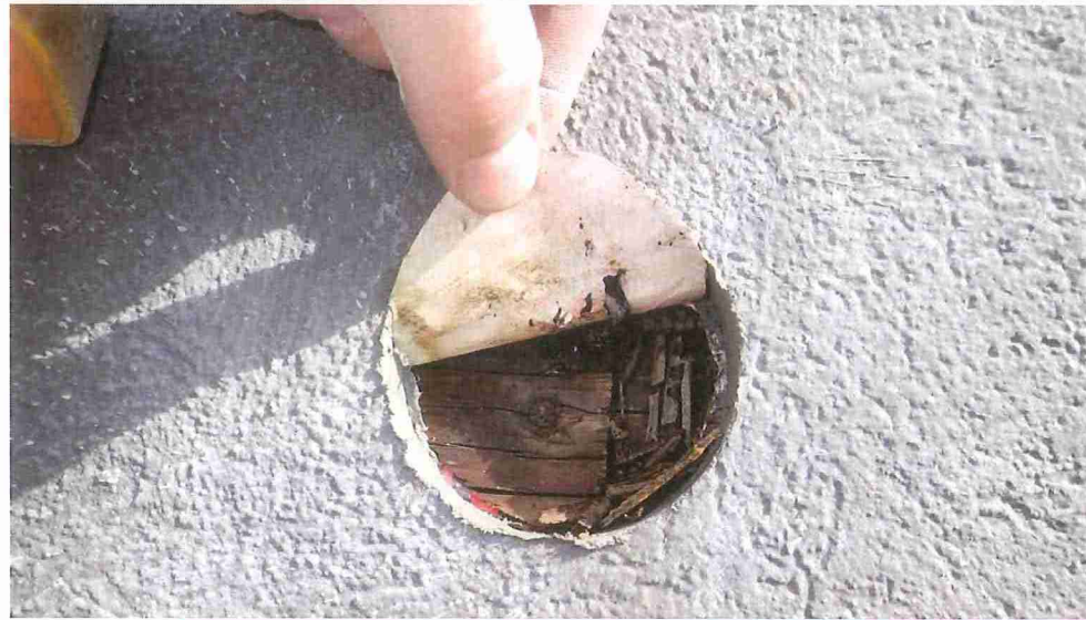
EXPLORAYORY OPENING #8 - SOUTH ELEVATION, WINDOW INTERFACE
