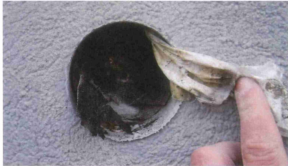
EXPLORAYORY OPENING #12 - WEST ELEVATION, WINDOW INTERFACE
