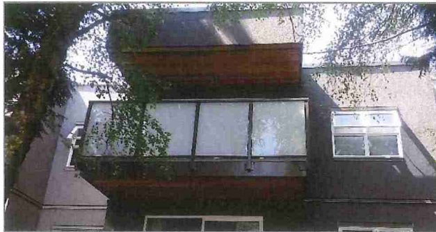
Figure 3.10 Aluminum-framed guardrail with opaque glass.
