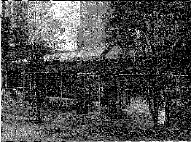
Front view of the Subject Strata Lots
